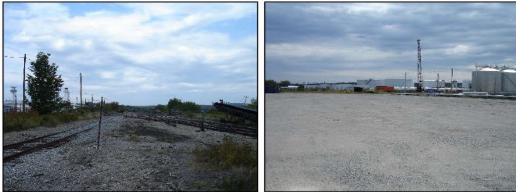
Figure 13: Existing Main Rail Yard and Heavy Weight Pad Area 75
